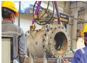
Valve Repairing / Replacement Services
