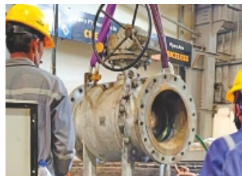
Valve Repairing / Replacement Services
