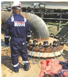
Bolt Tensioning Services
